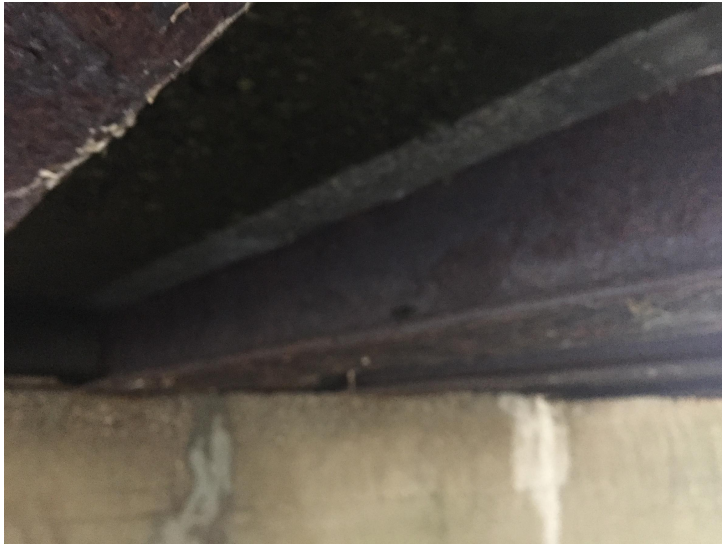
Document Name: IMG_0079.JPG Category: Superstructure Comments: Hole in web of beam 6w near south abutment
